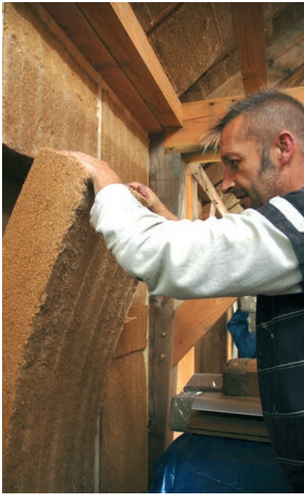
Previous page: timber-framed house insulated internally. This page: Wood fibre (left) and sheep's wool insulation are natural and breathable.
